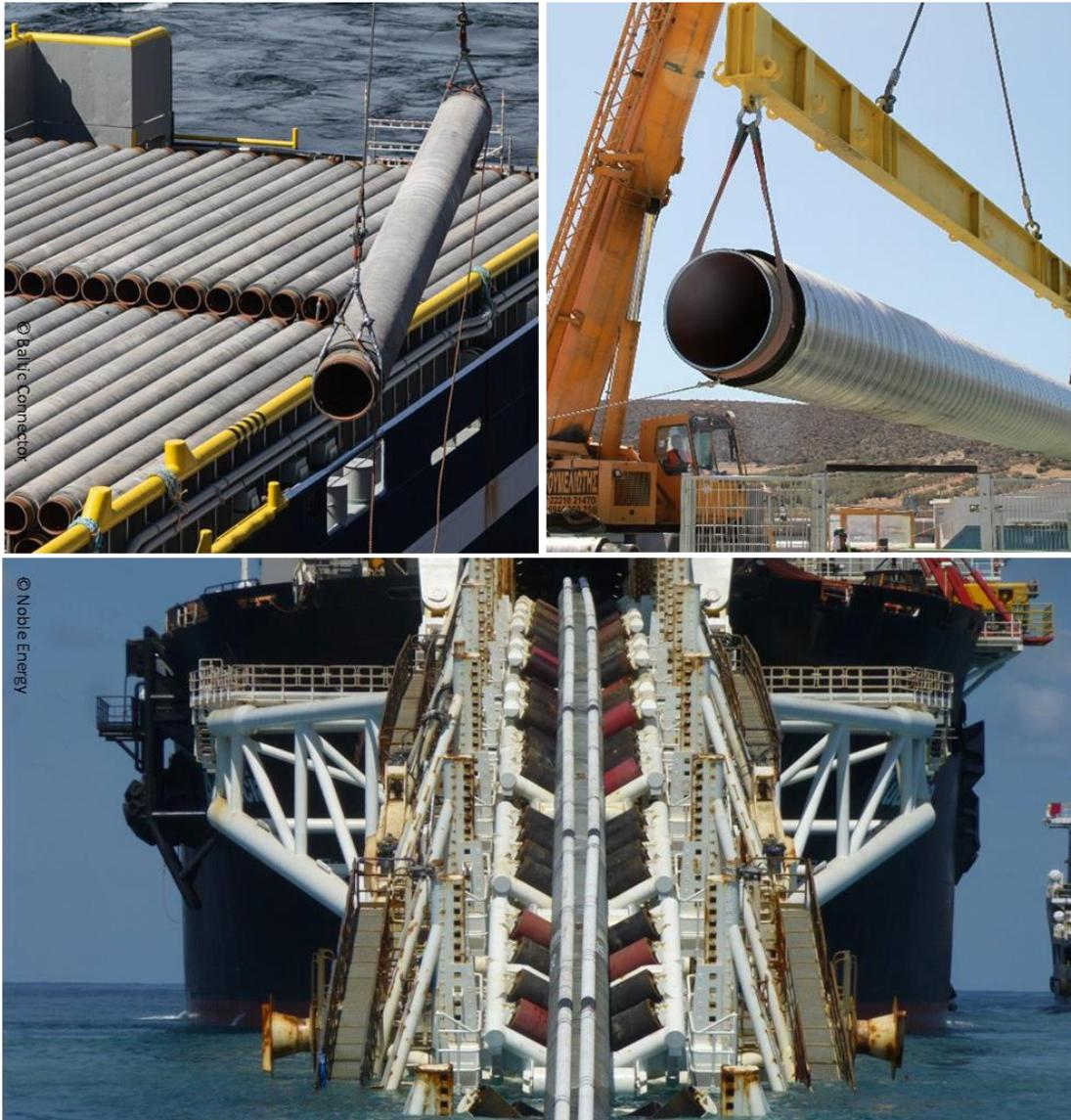
Image 1: Loading of CWC pipes to the laying vessel for Balticconnector project
