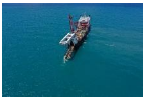
> Karish gas export pipeline SE Mediterranean Gas, Offshore deep (max 1.750m) 100 Km
