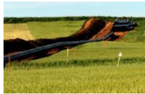
> Snam projects Italy, Gas, onshore >1.000km
