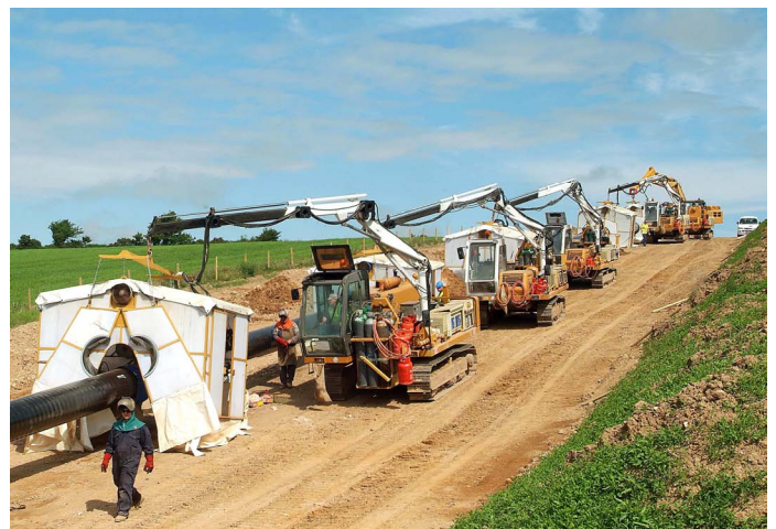
Figure 18: Mainline welding spread
