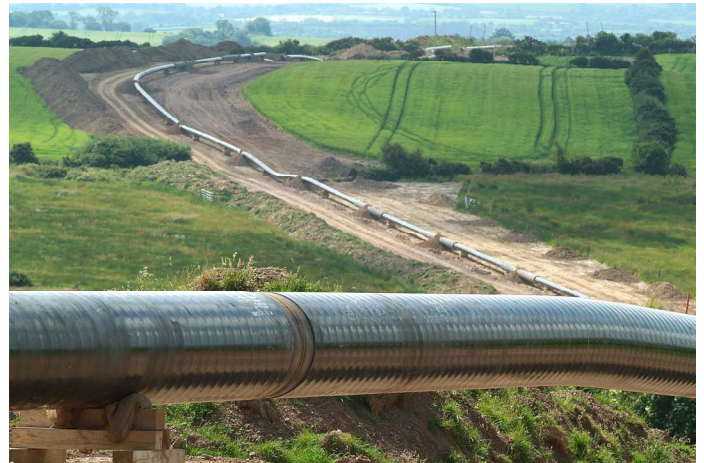
Figure 17: Curraleigh West to Midleton Pipeline – General view
